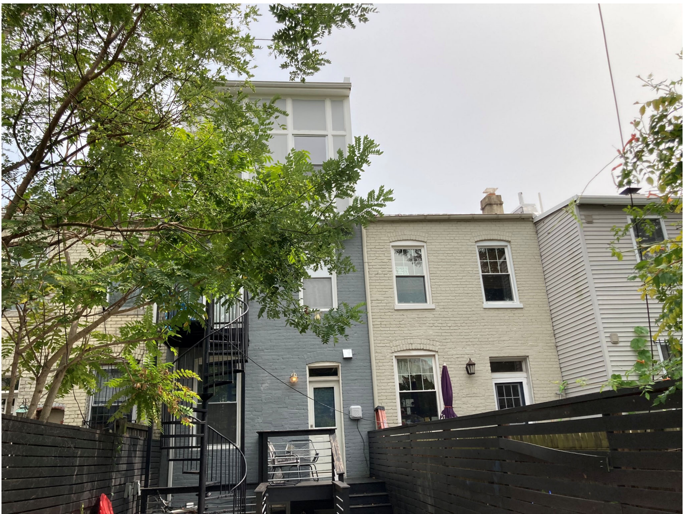
REAR ALLEY, HOUSES FRONTING 14 TH STREET SE
