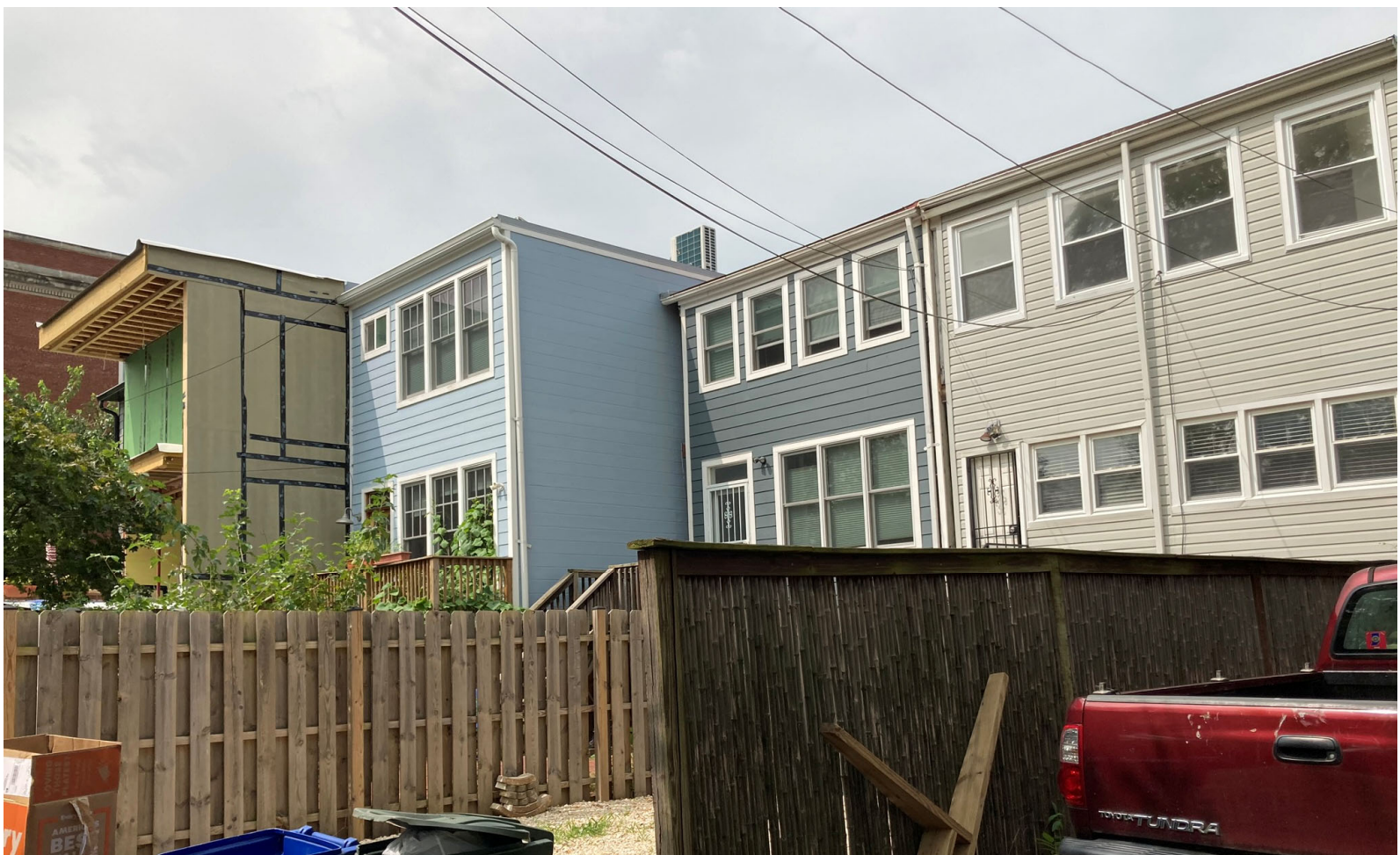
REAR ALLEY, LOOKING SOUTH-WEST
