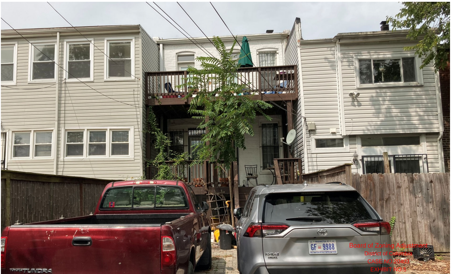
EXISTING REAR FACADE
