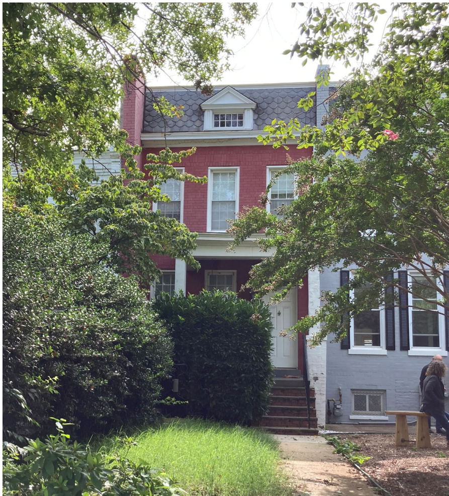
EXISTING FRONT FACADE
